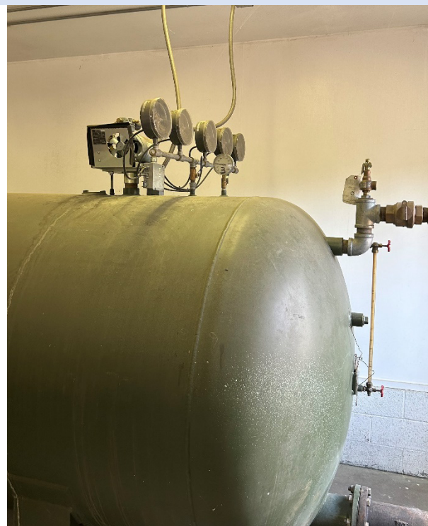
6-unit Pressure pump system with 10k pressure tank.
