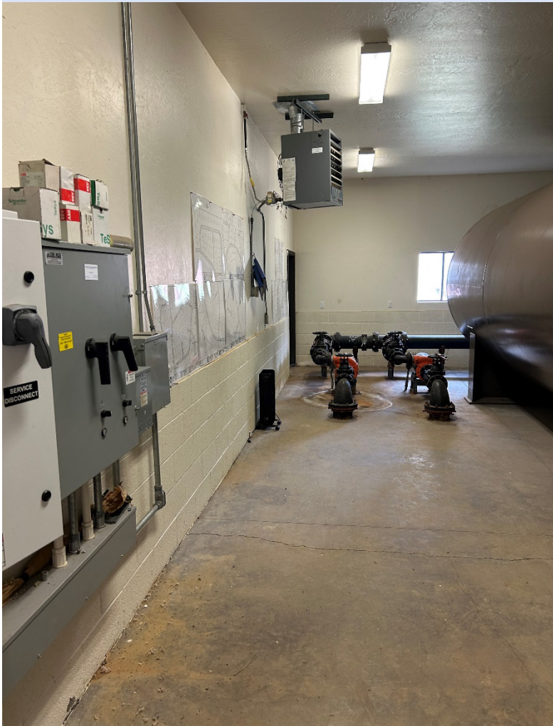
Pressure pump system with 10k pressure tank.
