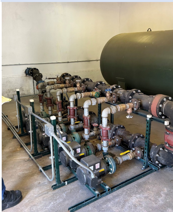
6-unit Pressure pump system with 10k pressure tank.
