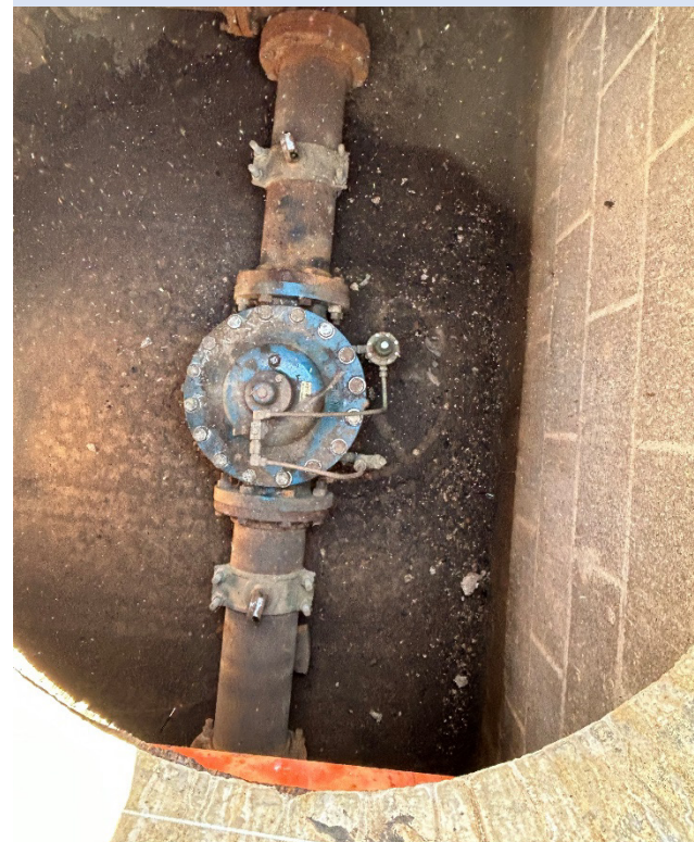
In-line Pressure Relief Valve
