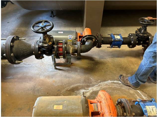
Pressure pump system with 10k pressure tank.
