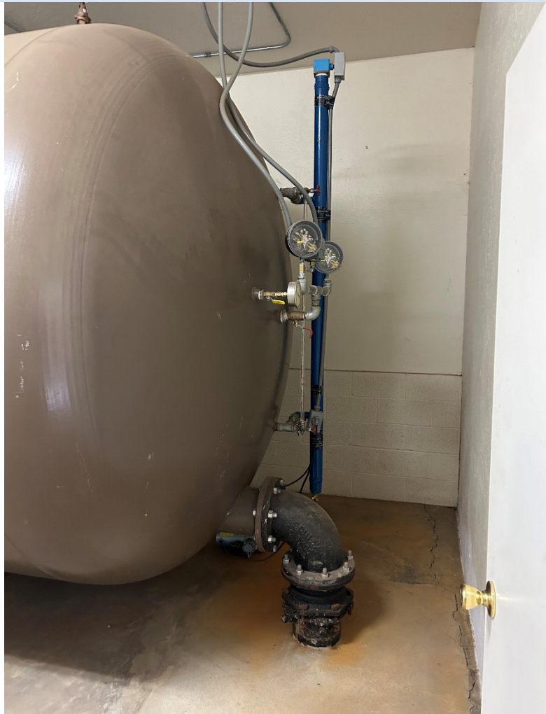
Pressure pump system with 10k pressure tank.
