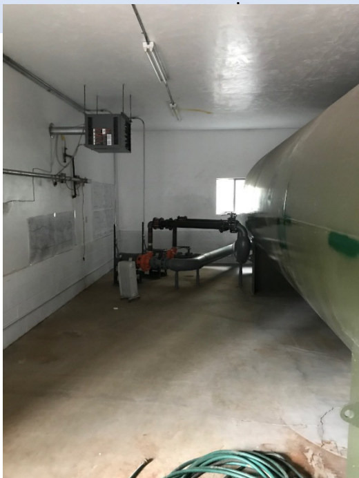
Pressure pump system with 10k
